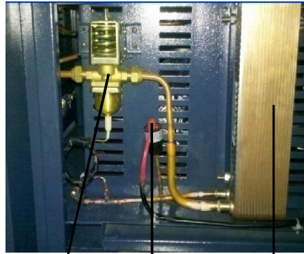
Water flow regulator Resettable pressure switch Brazed Plate exchanger (water-cooled condenser)
