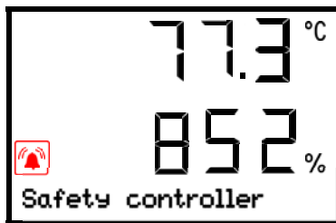
Normal display showing safety controller alarm (sample values)
